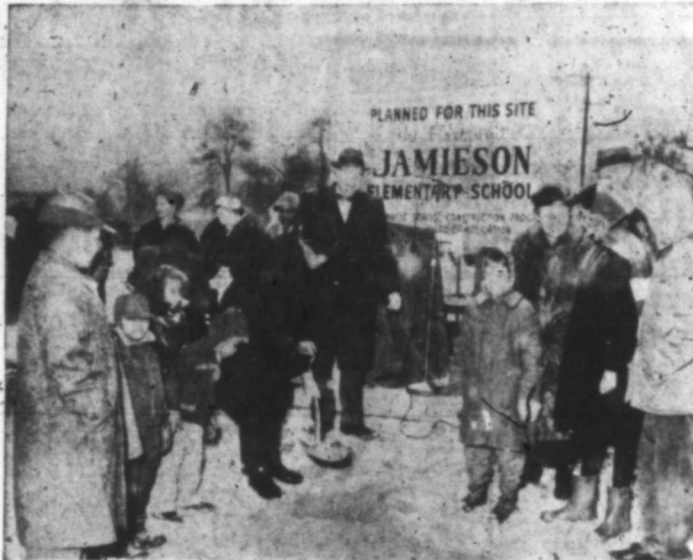
DR. REMUS G. ROBINSON, member of the Detroit Board of Education for the past six years and president of the board during the 1958-59 school year, breaks ground for the new Jamieson Elementary School at 2900 W. Philadelphia. The first
