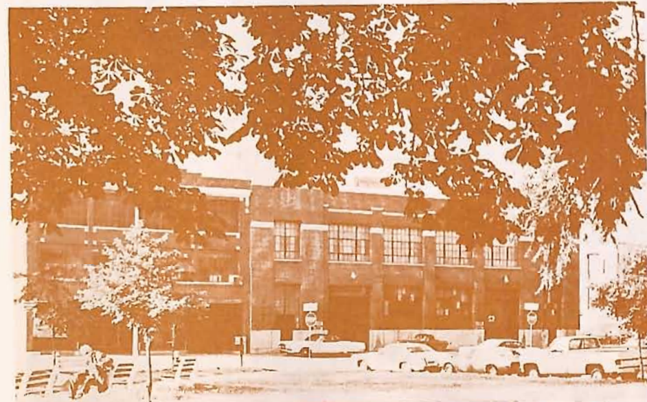
The driveway of the Detroit Edison Company's Garage on Ledyard Street where Clarence Manning Jr. was killed by STRESS.
